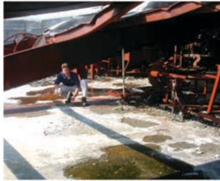
Spalling in manufacturing facility exposed to fire.
